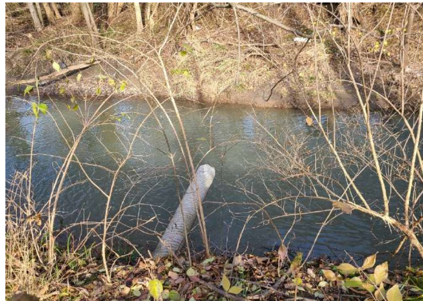
8. A pipe entering Tontogany Creek near NW corner of the Site. May drain neighbors' property or part of the Site.
