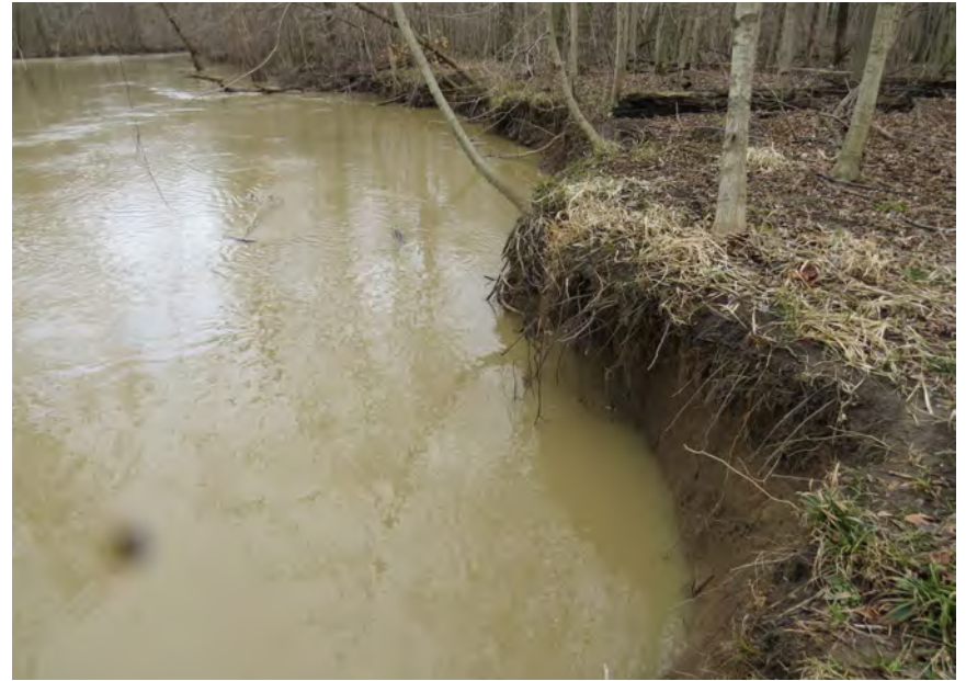
6. Erosion along bank of St. Joseph River.
